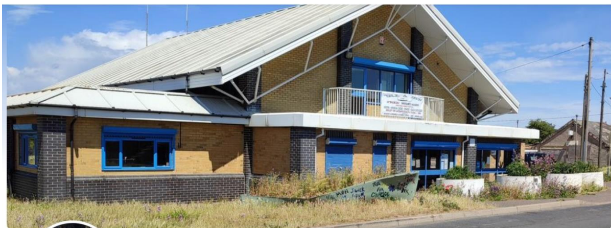
Community and Resource Centre, Jaywick
